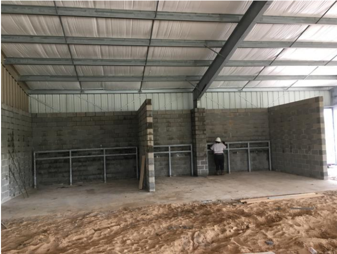
1. CMU partitions at large animal wash downs
