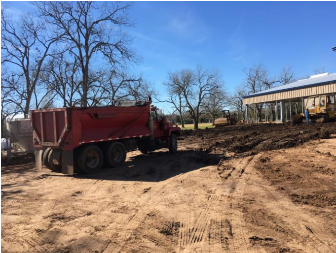
3. Import of soils for required elevation
