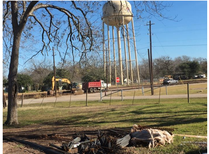
4. Excavation of mitigation pond
