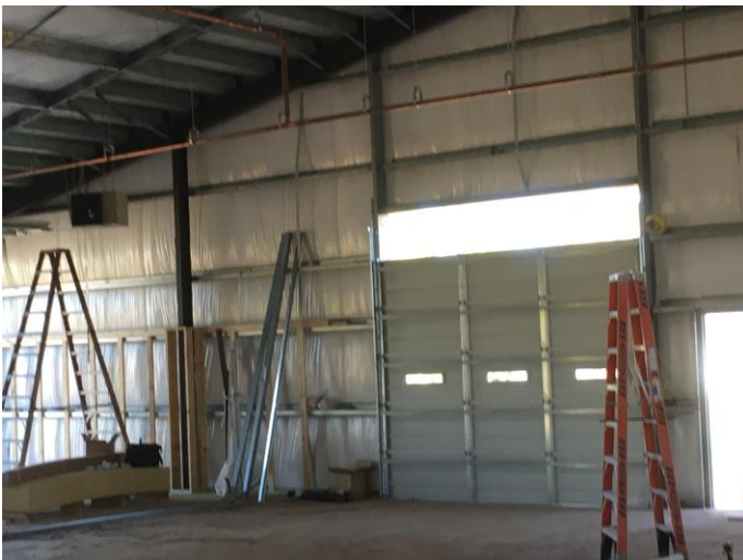
5. Installation of overhead doors
