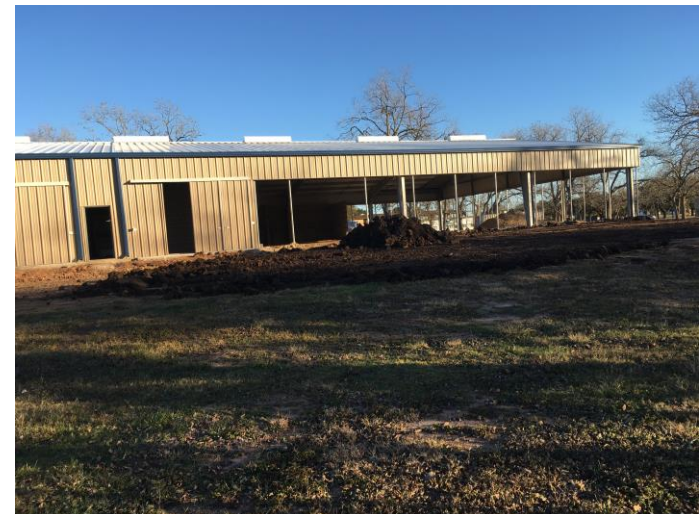
6. Import of soils for required elevation
