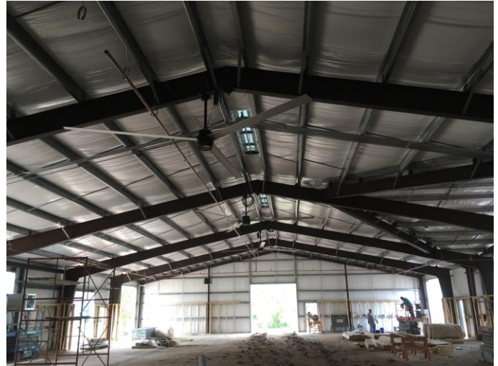
2. HVLS fan installation at small animal area
